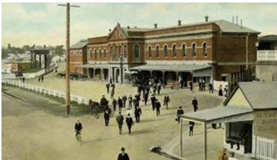
Opening of South Brisbane Station 1891
